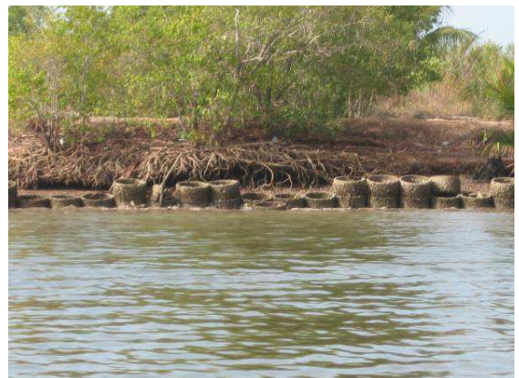
This two photos show adaptation approaches of community in Krabi River Estuary. To slow down coastal erosion , some community use concrete drain pipes , other use bamboo stakes.
