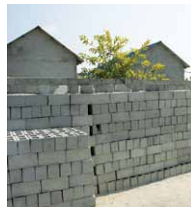
The waste management centre under construction on Vaikaradhoo Island, Maldives © Hanying Li
