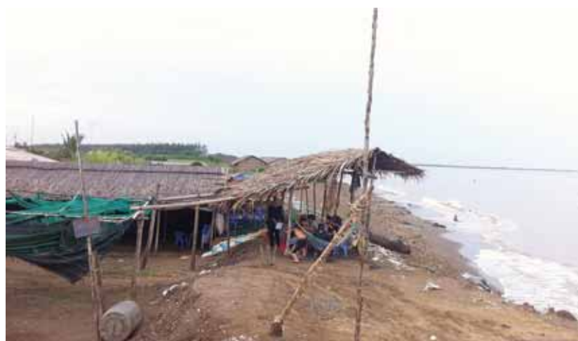
Figure 2: Simple stilt houses constructed onshore as restaurants and coffee shops to welcome local tourists on Bao Thuan coast. Ben Tre, Vietnam, Phong Nguyen, IUCN Ben Tre Project 2014
