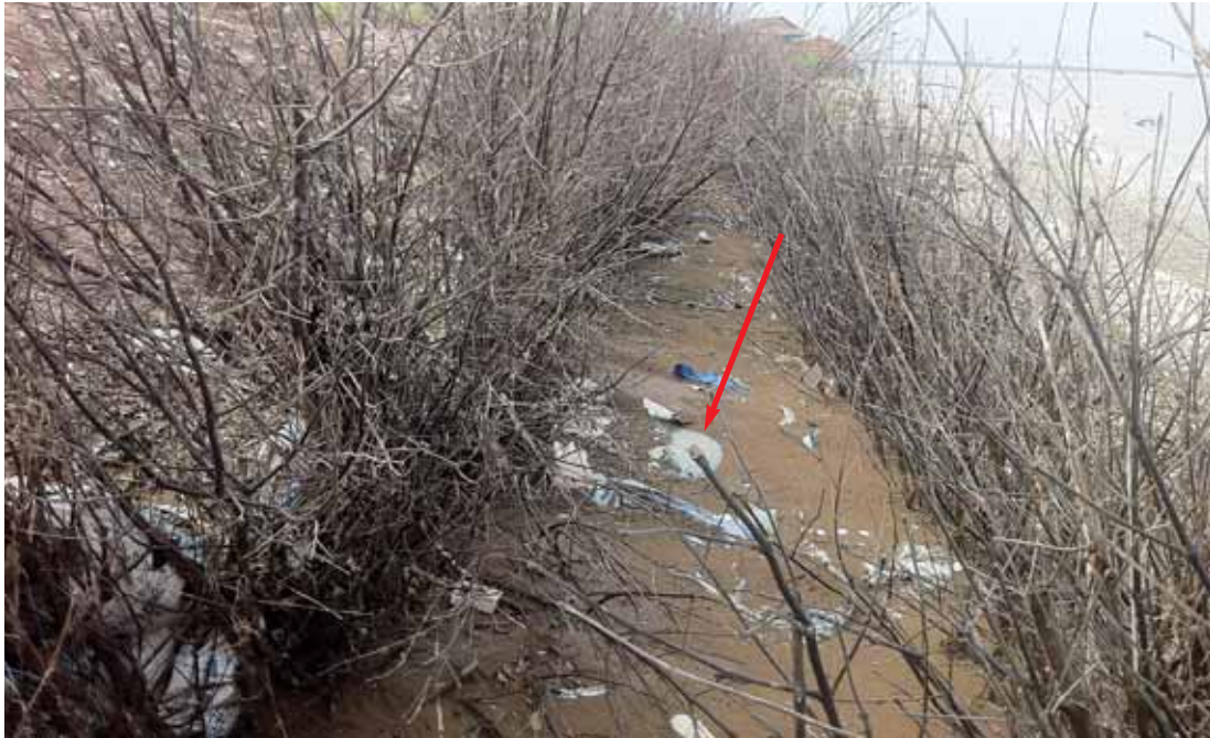
Figure 28: Double brush fences were reinforced by using sand bags placed between two lines of dried brushes of Rhizophora apiculata to protect agricultural land in Bao Thuan commune, Ba Tri District. Ben Tre, Vietnam, Phong Nguyen, IUCN Ben Tre Project, 2014
