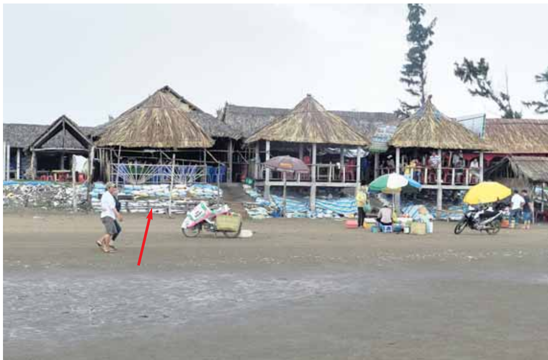
Figure 26: Bags filled with sand were piled up to construct fences to protect restaurants from erosion on Con Bung coast, Thanh Hai commune, Thanh Phu District. Ben Tre, Vietnam, Phong Nguyen, IUCN Ben Tre Project, 2014
