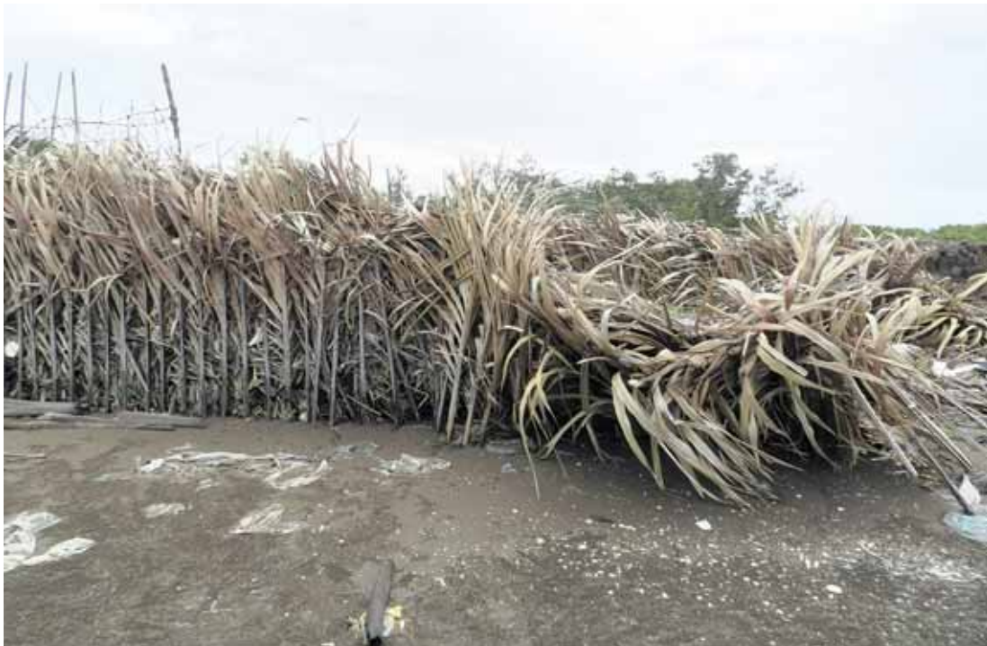
Figure 22: Nypa palm fence was weighed down by strong waves in high tides on Den Chop Area, An Thuy Commune. Ben Tre, Vietnam, Phong Nguyen, IUCN Ben Tre Project, 2014
