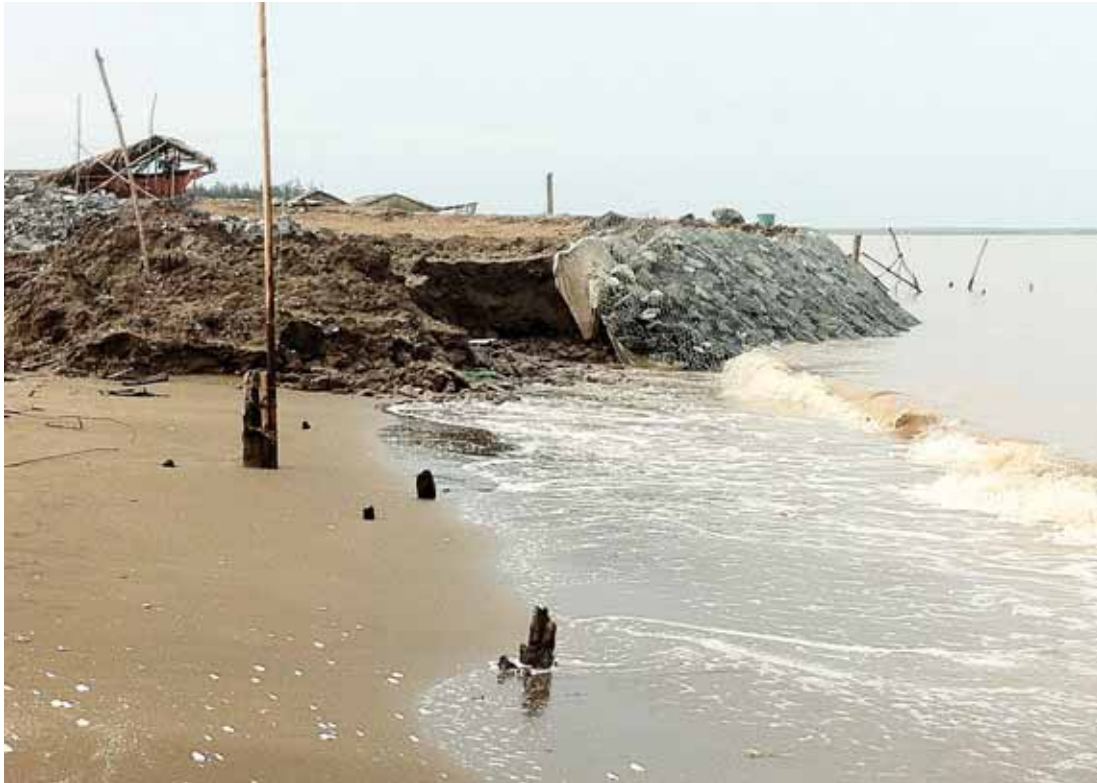
Figure 24: Simply constructed but expensive gabion revetments are unsure in protecting local properties in Bao Thuan commune, Ba Tri District. Ben Tre, Vietnam, Phong Nguyen, IUCN Ben Tre Project, 2014
