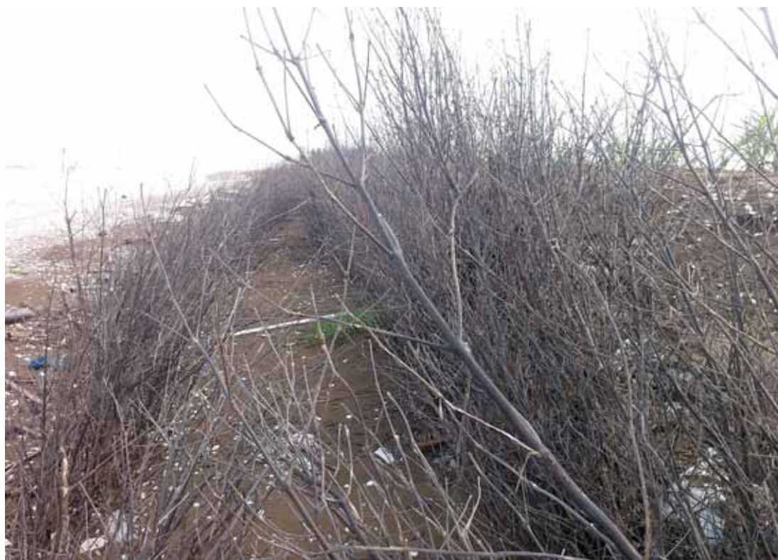
Figure 27: Fences constructed by using two lines of dried brushes of Rhizophora apiculata to protect agricultural land in Bao Thuan commune, Ba Tri District. Ben Tre, Vietnam, Phong Nguyen, IUCN Ben Tre Project, 2014
