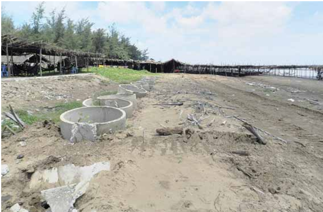
Figure 23: Broken and sunk concrete piles were seen ineffective in protecting local restaurants on Cong Be Lon area, Thua Duc commune, Binh Dai District. Ben Tre, Vietnam, Phong Nguyen, IUCN Ben Tre Project, 2014
