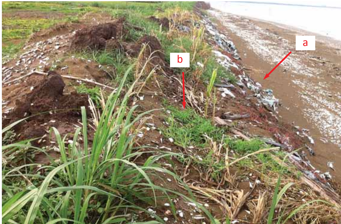
Figure 25: The photo showing sand bag fences, a) sand bag piled up to construct a fence, b) grasses were grown on topsoil behind the sand bags to reinforce the fence in Bao Thuan area. Ben Tre, Vietnam, Phong Nguyen, IUCN Ben Tre Project, 2014
