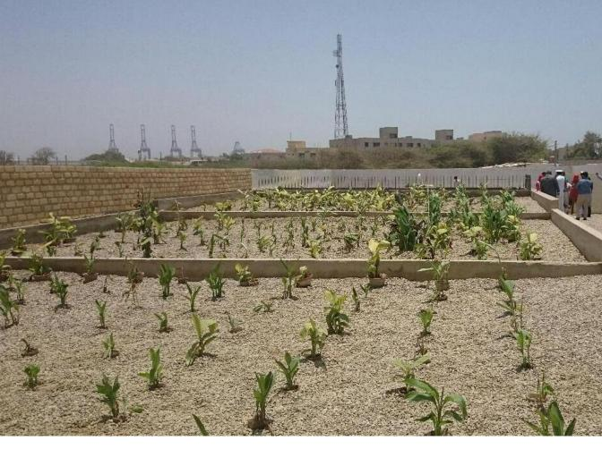
designed to imitate the processes found in natural wetland ecosystems. The system involves a series of gravel filter beds planted with reeds to treat wastewater passing through the root zone. The system is cost-effective as it is less energy-intensive than traditional wastewater treatment techniques and uses natural materials and processes. The project has helped in saving thousands of gallons of freshwater that may otherwise have been used for the greening purposes.
