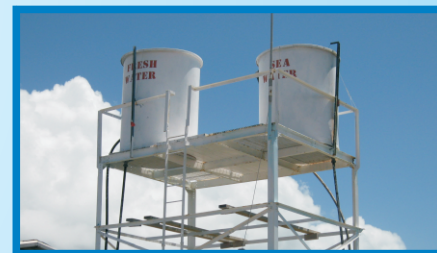
Water tower - 1 salt water tank, 1 fresh water tank
